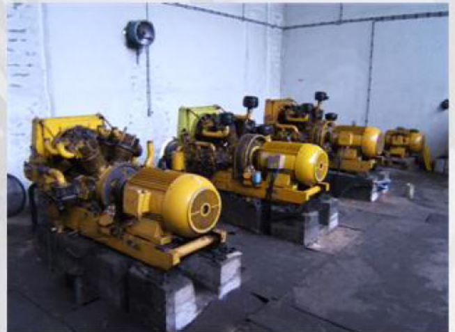
Name: Fagor – Smederevo Type: KS – 707 – 2 Manufacture: OOOR – Inzenjering Smederevo Capacity 25 m 3 /min Compressor ES 707 – 2 Work pressure 9 atm. Year of production 1981 Number of compressors: 4
